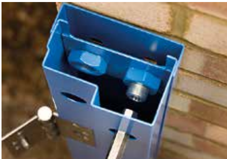
STEP 2: Ensure you have a square and tight frame using the adjuster screws.
