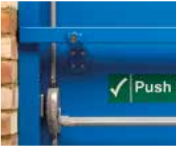
Lockable drop bar complete with pinson locks.
