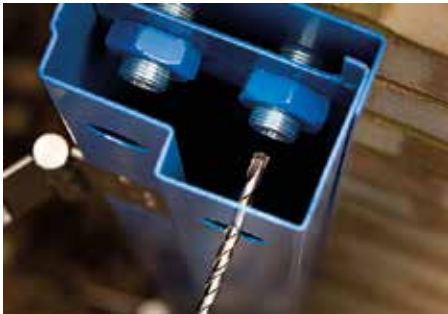
STEP 3: Once the frame is in position, drill through the frame adjuster screws.
