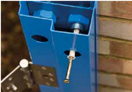
STEP 4: Insert the frame fixers.
